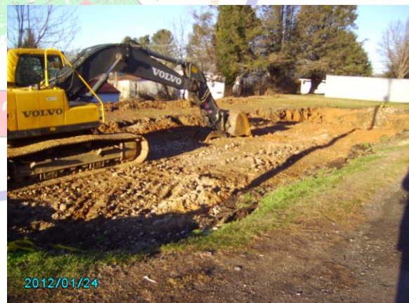
Ag bldg site and debris removal
