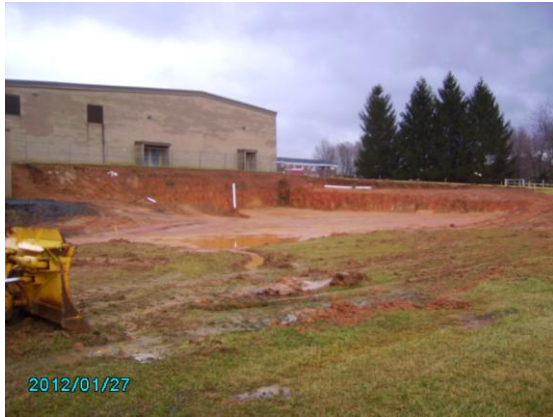
Building pad where unsuitable soils have been removed.
