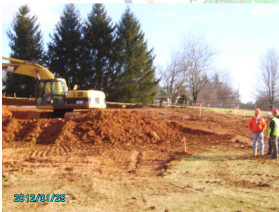
Removal of unsuitable soils from Classroom building pad
